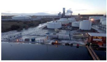
ABOVE: InterTerminals, RiversideTerminal. Water overtopping the flood defences – as seen from a ship at the terminal. BELOW: SABIC Brinefields and Cavities storage area showing the flood defence breach. © Environment Agency
